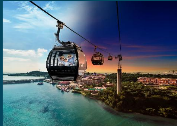
Monocablable Detachable Ropeway Location: Panjim & Reis Magos Ropeway Capacity: 800 PPH (upgradable to 1000 PPH) Length of the Ropeway facility: 1240 m.
